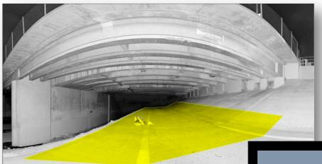
Measured clearance at the damage location is around 12 feet
